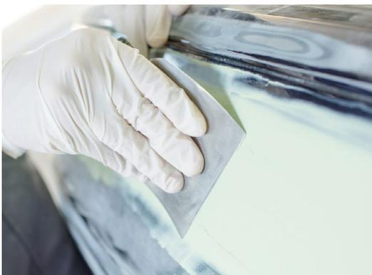
Apply a uniform layer of "Marble Putty" on the prepared surface, using a putty knife to ensure uniform distribution of the product on the surface of the marble.
